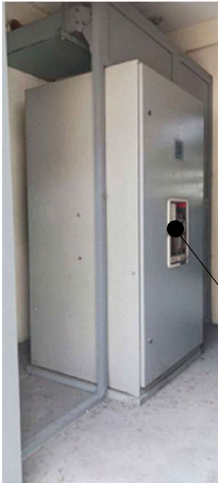
MAIN AIR CIRCUIT BREAKER (FRONT VIEW)
