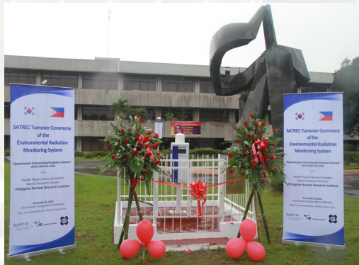
Top: The EFRD-3300 Environmental Radiation Monitoring System
