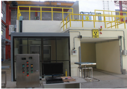
Top: The electron beam facility in its final stages of construction
