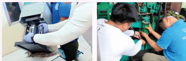
Preventive maintenance activities at CTBTO PHP52 station such as hydraulic fluid refill of the hydraulic press (left), oil filter cleaning of generator set (center), and air filter change for air sampler intake sphere (top)
