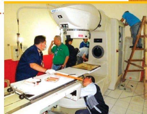
Decommissioning of Cobalt-60 teletherapy at Baguio General Hospital and Medical Center
