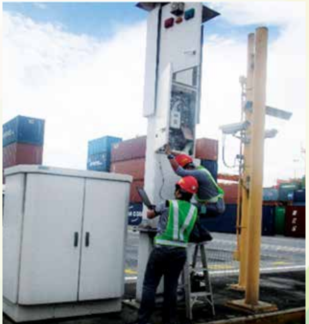
Troubleshooting of radiation portal monitors at the South Harbor in Manila
