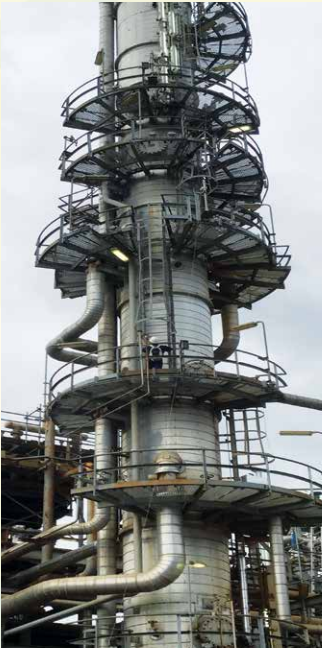
PNRI performs gamma column scanning to test the operating conditions of a distillation column in a refinery.
